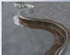
Top waterproofed with TexTop .
