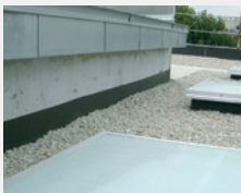
Upstand waterproofed with TexTop .
