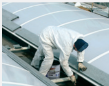
Gutter waterproofed with TexTop .
